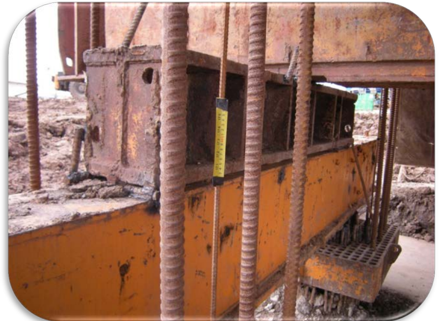
Anchor Pile Uplift Measurement
